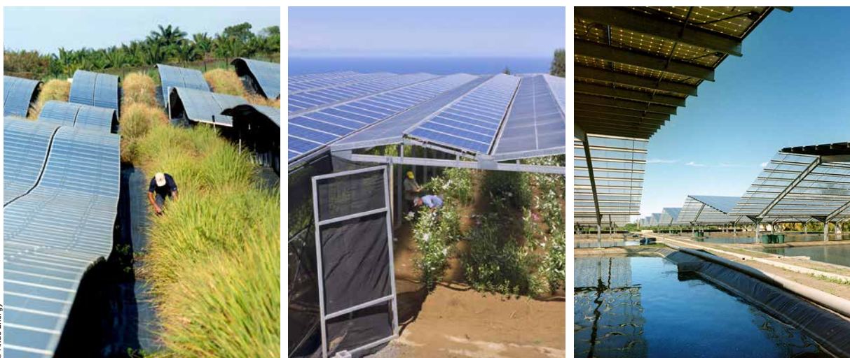
The first and second generation of 'Agrinerjie', and the 'Aquanergie' solution covering fish farms.
